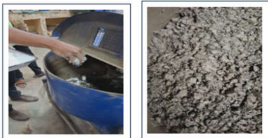
Fig.4.2 Mixing of Concrete
